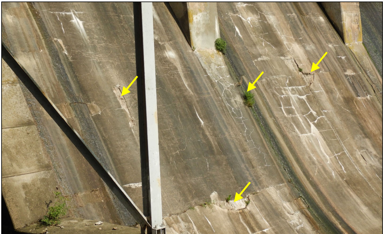
Photo 4 – Concrete deteriorations on the downstream face and the toe of the Spillway bays
