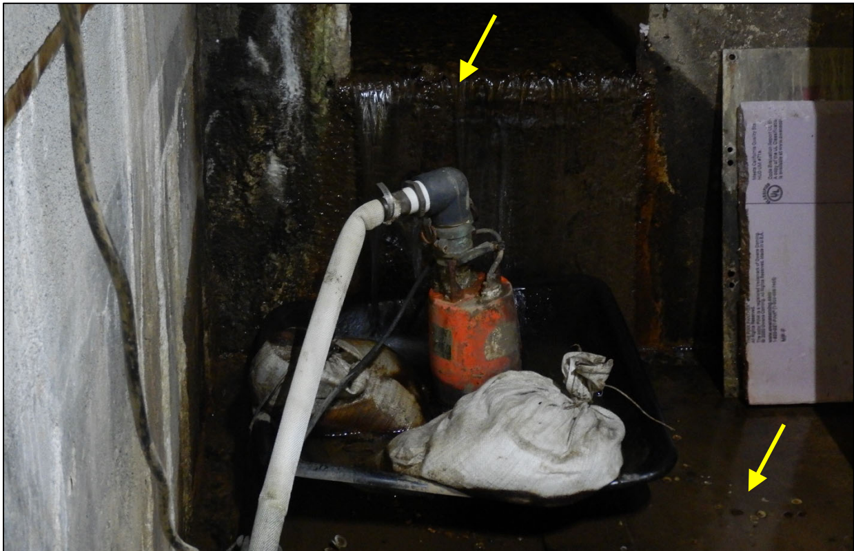
Photo 9 – Seepage with ponded water in the confined space behind Units 8 to 11 (it is being collected and pumped into a drain, but the floor is slightly ponded)
