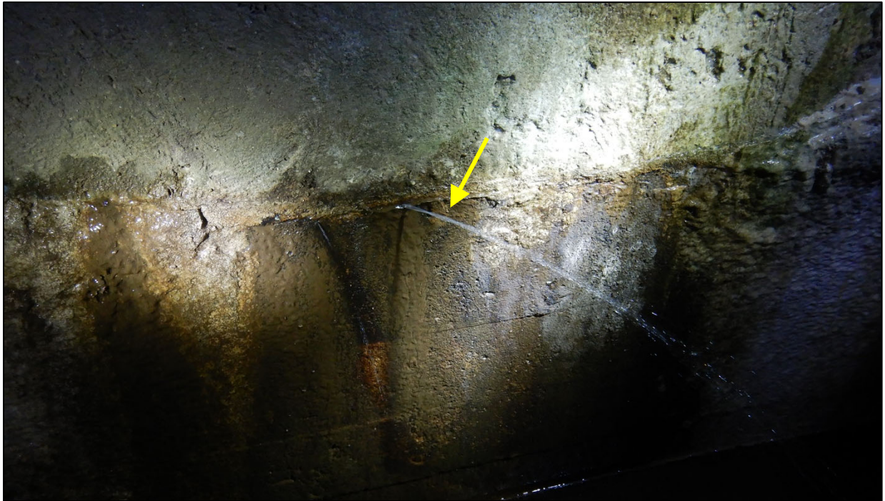
Photo 8 – Leakage from the upstream wall of the inspection gallery in the vicinity of Crest Gate 21
