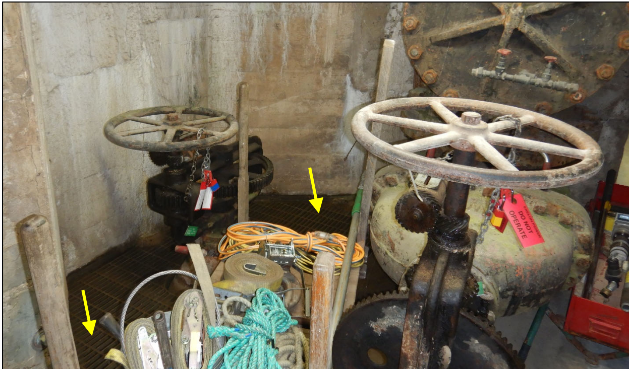
Photo 11 – Ponded water by the Unit 2 controls in the powerhouse inspection tunnel
