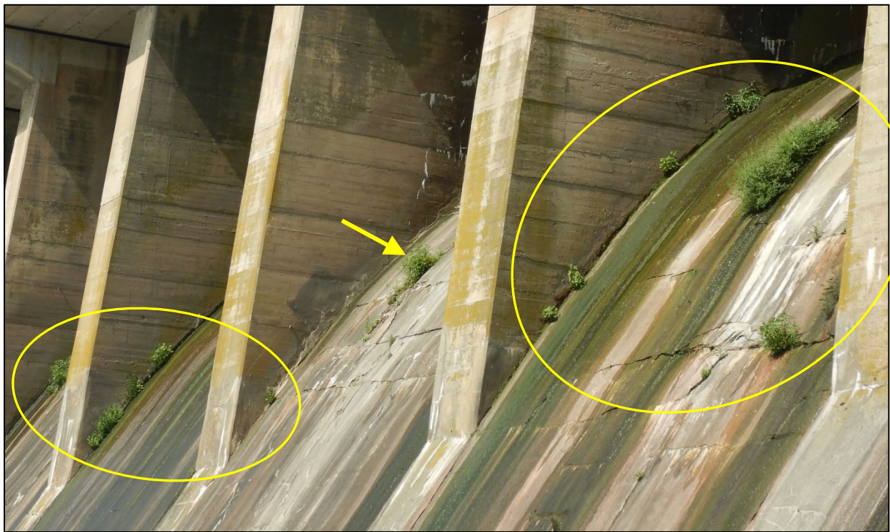
Photo 6 – Vegetation growing from the cracks / deteriorations on the downstream face of the Spillway bays
