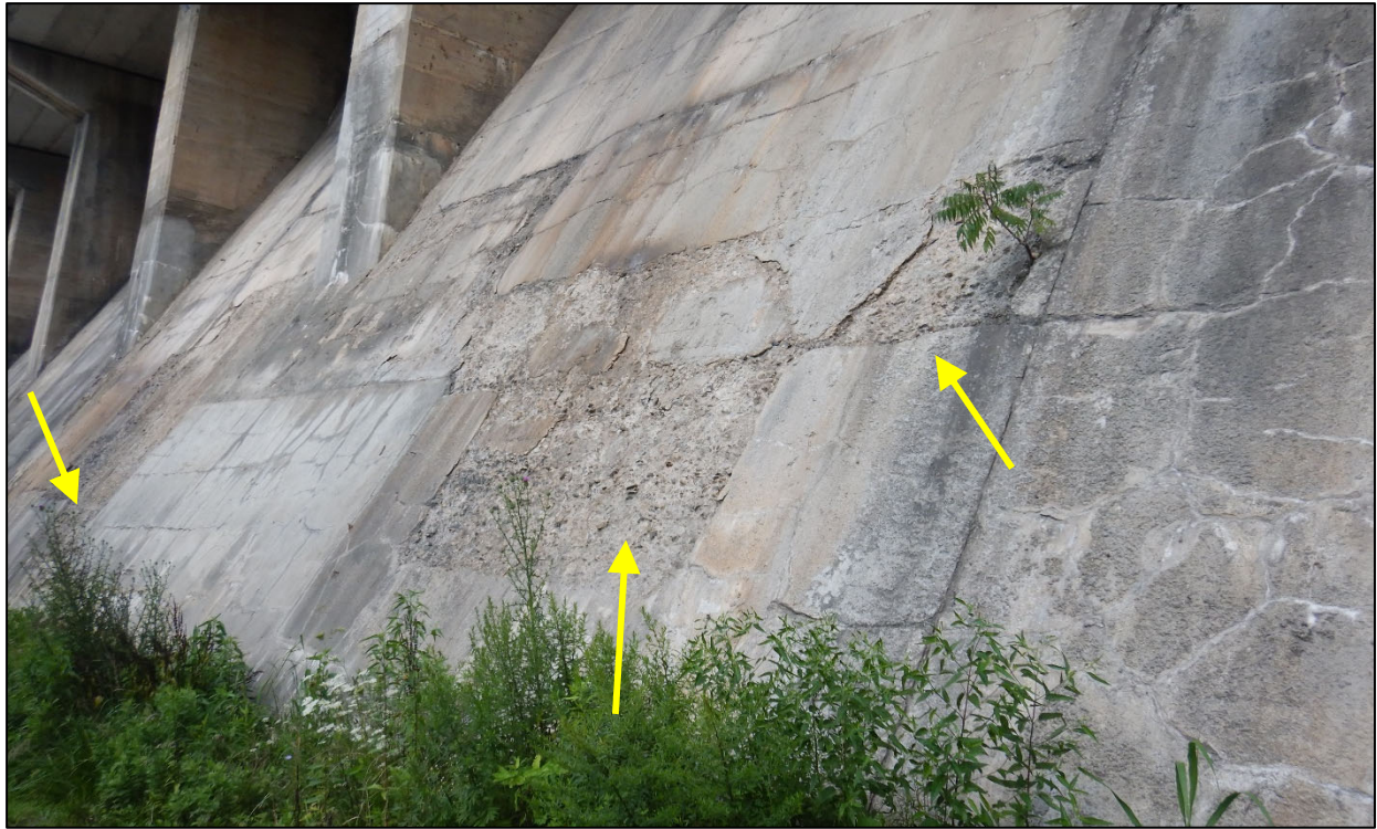
Photo 5 – Concrete deteriorations on the downstream face of the Left Non-Overflow section
