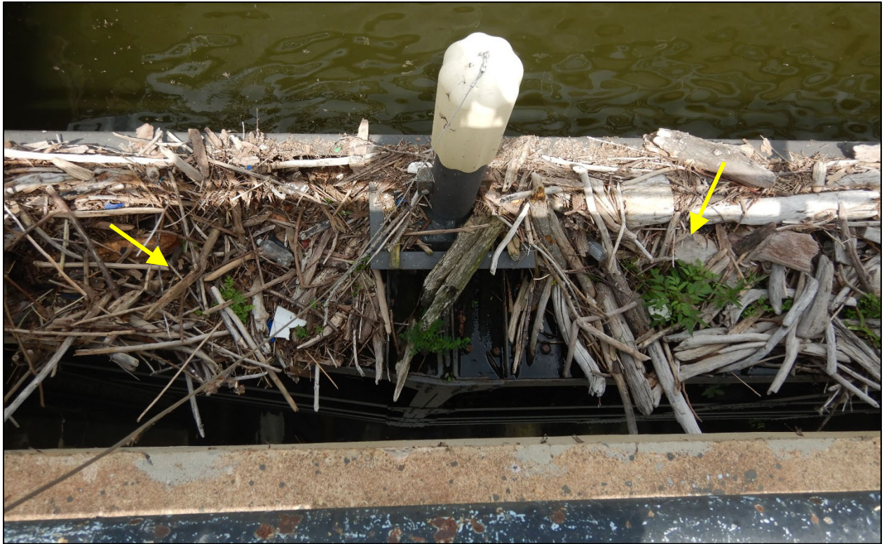
Photo 1 – Deposit of debris and vegetation on a few of the Spillway gates
