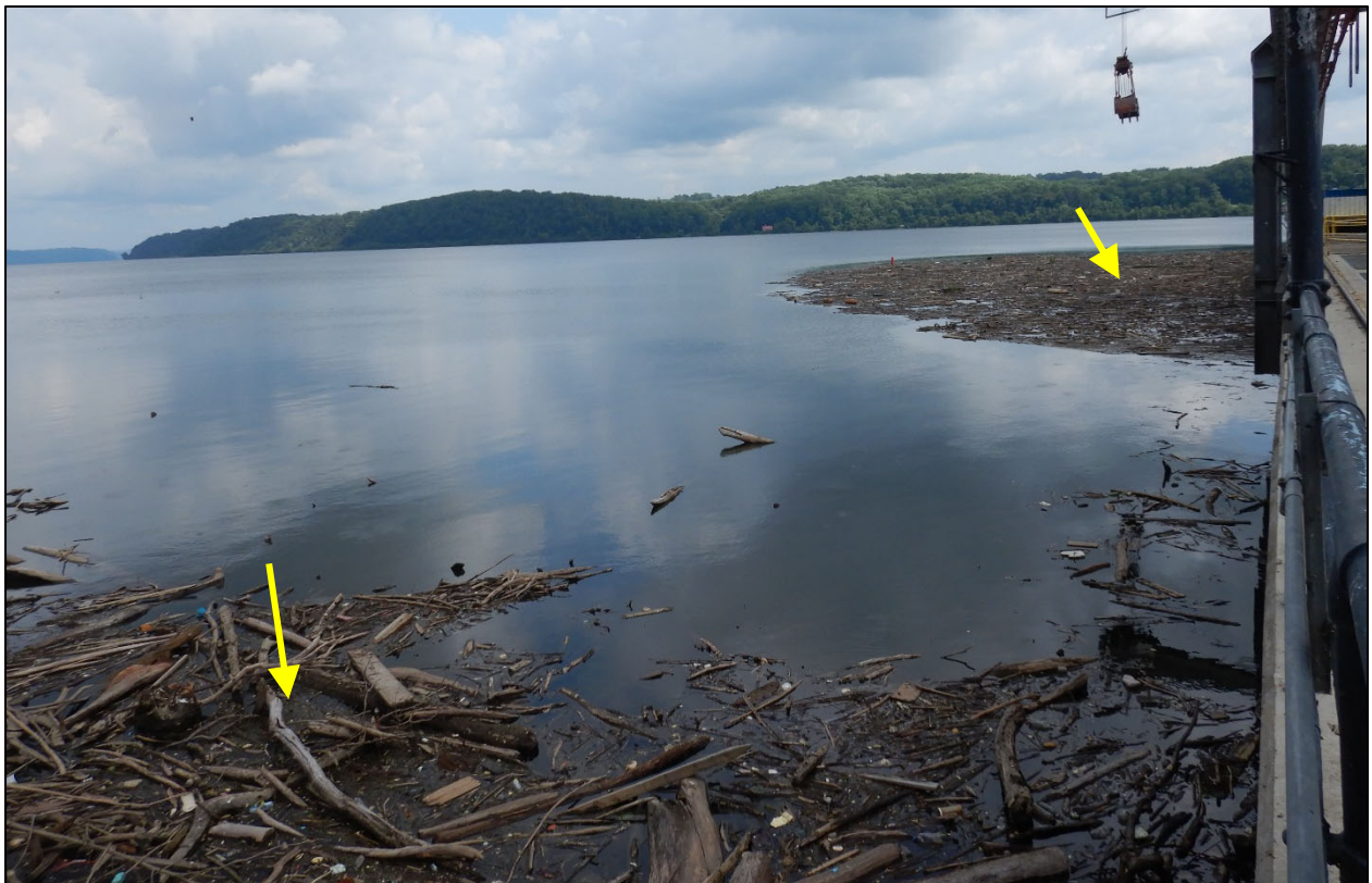
Photo 2 – Debris on the upstream side of the Powerhouse Intakes and the Spillway gates
