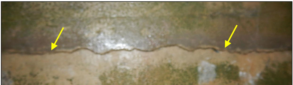
Photo 7 – Cracks on the downstream and upstream walls of the inspection gallery
