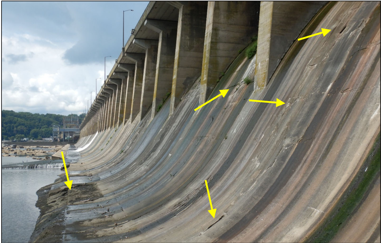
Photo 3 – Concrete deteriorations on the downstream face and the toe of the Spillway bays
