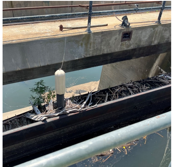
Photo 1 – Deposit of debris and vegetation in the spillway gate structures (found in most of them)
