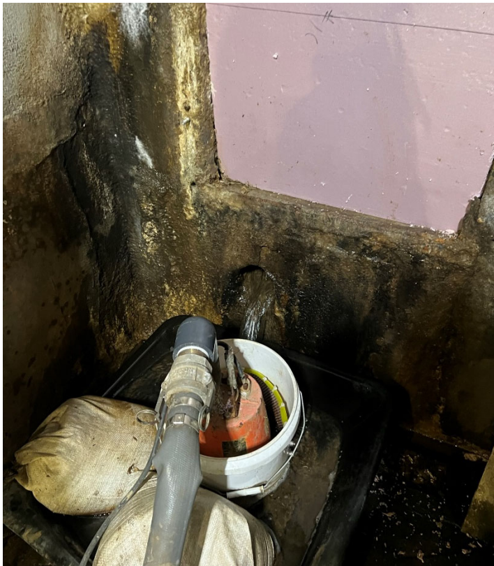
Photo 2 – Seepage in the confined space behind Units 8 to 11 being collected and pumped into a drain
