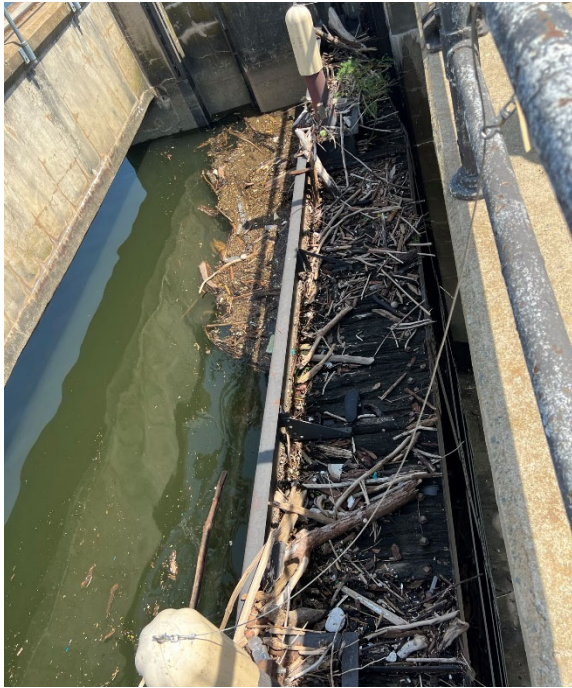
Photo 1 – Deposit of debris and vegetation in the spillway gate structures (found in most of them)
